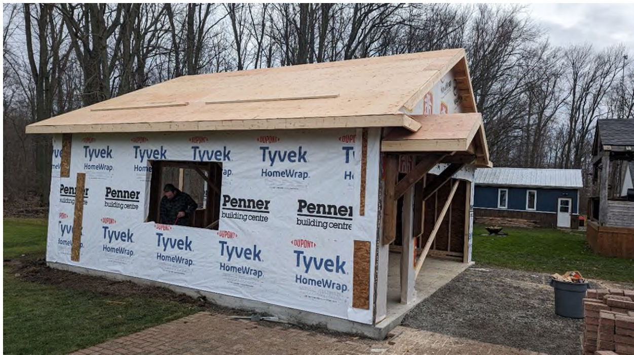
Figure 3 - Accessory Structure Under Construction
