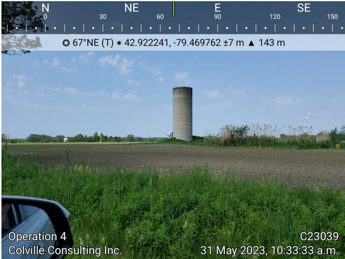
Photo 9: Operation #4 – Remnant farm showing uncapped cement silo.
