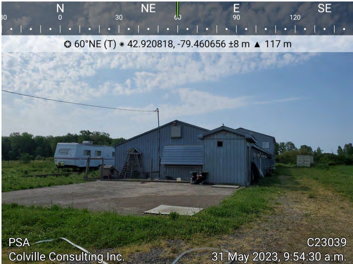
Photo 2: Operation #1 – Small chicken coupe and agricultural building used for storage located within Subject Lands
